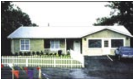
Attractive ranch home model built with the First National Panel System.
